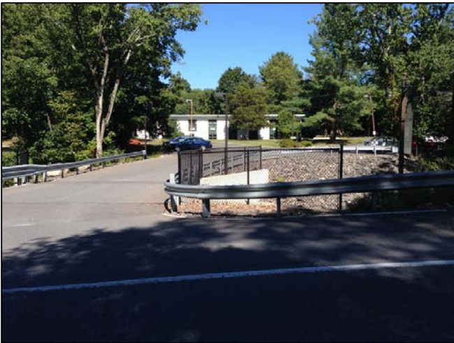
RETIREMENT COMMUNITY – VIEW OF ACCESS DRIVE WITH BRIDGE HARDENED AFTER IT BLEW-OUT TO A STORM EVENT (CREDIT: TETRA TECH)
