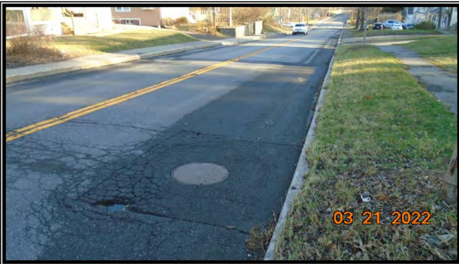
**Photo No. 4** – Photo looking northerly on South Chestnut Street (Route 208) Note patch where recent sewer collapse occurred)
