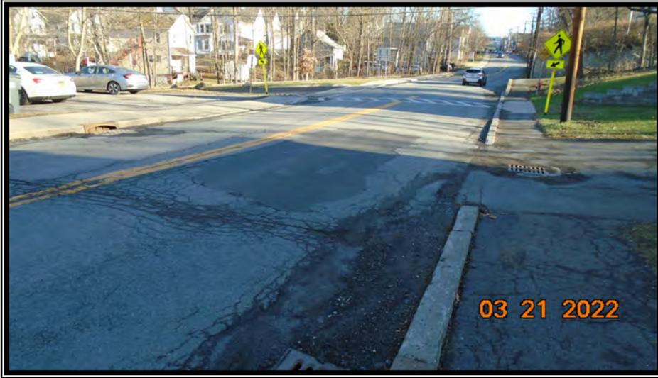
**Photo No. 7** – Photo looking northerly on South Chestnut Street (Route 208) Note patch where recent additional sewer collapse occurred)
