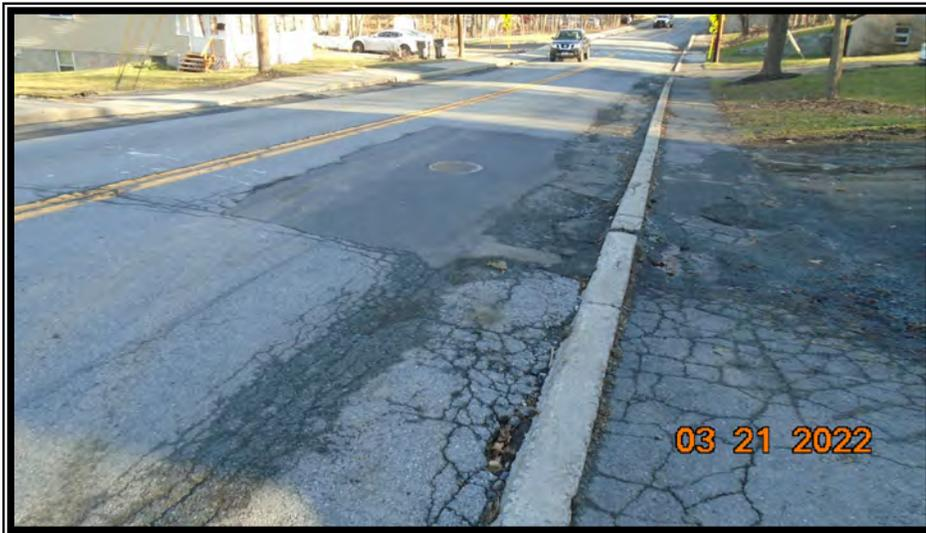
**Photo No. 6** – Photo looking northerly on South Chestnut Street (Route 208) Note patch where recent additional sewer collapse occurred)
